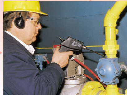
Ultraprobe 100 testing pump valve leaks
