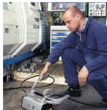
Lifting a machine with a cylinder and air hydraulic pump with remote control.
