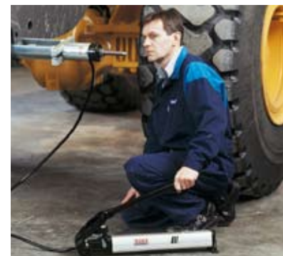
Replacement of a bushing using a hollow cylinder and hand pump.
