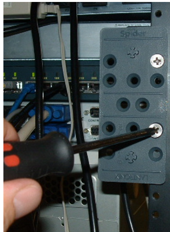
Figure D-2 Attaching the Mounting Bracket
